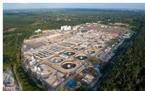
Czajka Wastewater Treatment Plant, POL
