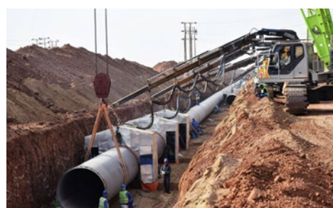
Ras Al Khair-Riyadh Water Transmission System, KSA
