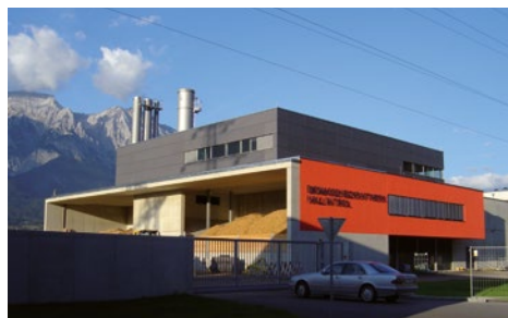
Hall Biomass-Fired Cogeneration Plant, AUT
