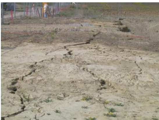
Figure 1: Tunnelling in near-surface rock conditions causing cracks and “cave-ins”
