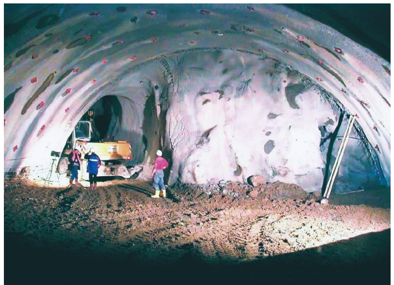
Fig. 4 Tunnel excavation in karst – Irlahüll tunnel.
