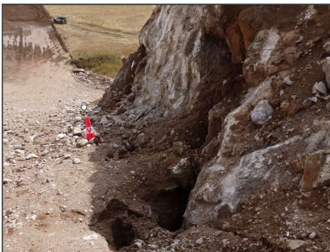
Figure 9: Large cave on the right of way after grading works (left) and after it had been opened (right)
