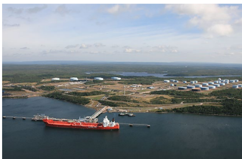
Green Ammonia Project, Canada
