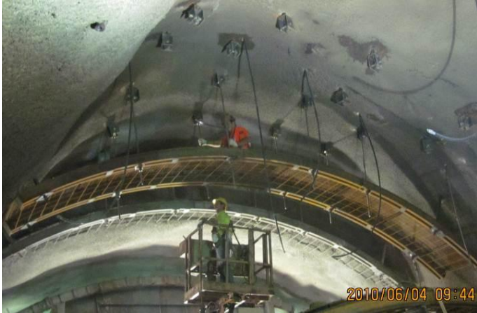
Figure 5. Installation of fill of overbreak Type 2
