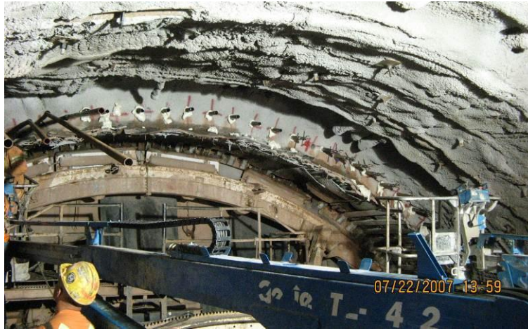
Figure 3. Spiling in area with overbreak, Support Type 4S
