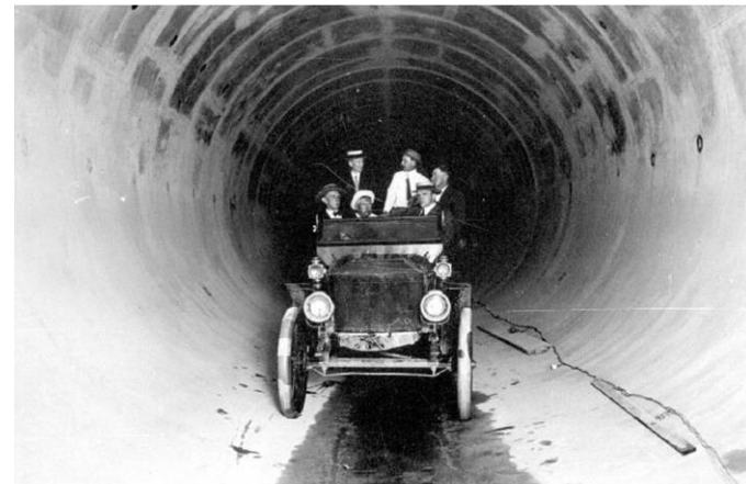
Ontario Power Conduit 2 Final Inspection 1905
