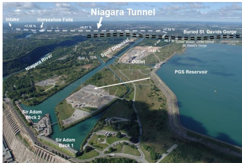
Figure 1: overview of the alignment of the Niagara Tunnel and Sir Adam Beck Station
