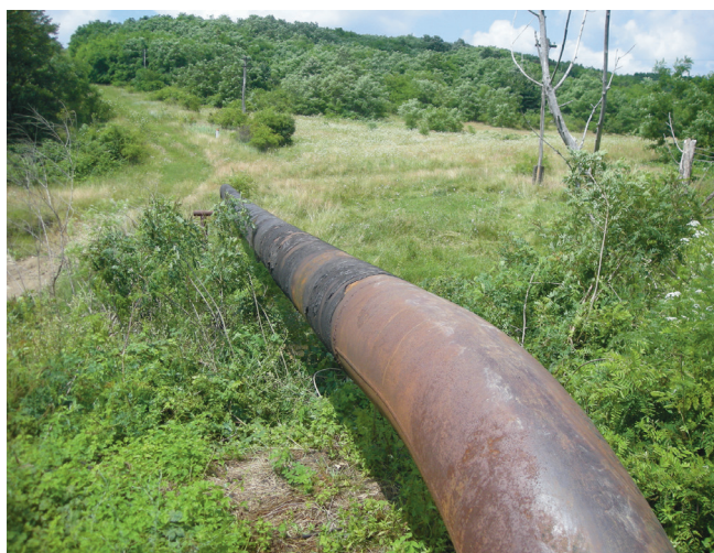
Figure 1. Coating condition.
