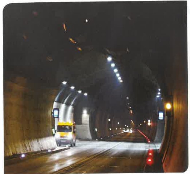
Illustration 2 - Lay-by in an Austrian motorway tunnel © ASFNAG
