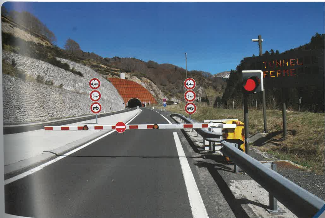
Illustration 6 - Effective tunnel closure enforced by barriers, Lioran Tunnel (France) © CETU
