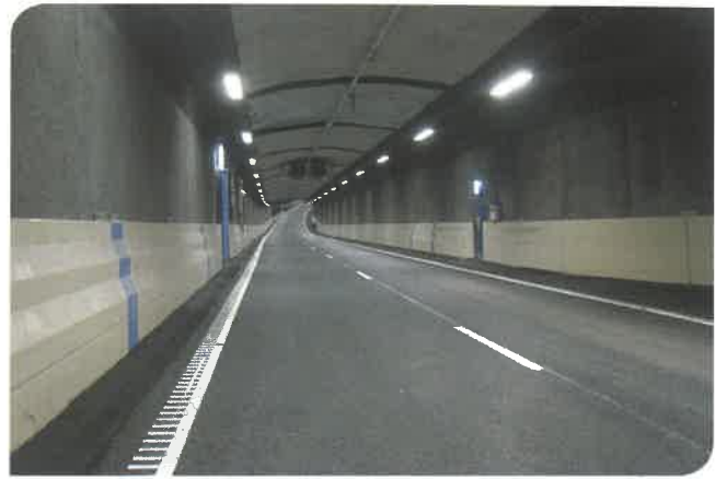
Illustration 5 - Tunnel cross section with lane marking by rumble strips and traffic guidance barriers on tunnel walls - Norra Länken Tunnel (Stockholm) © ILF
